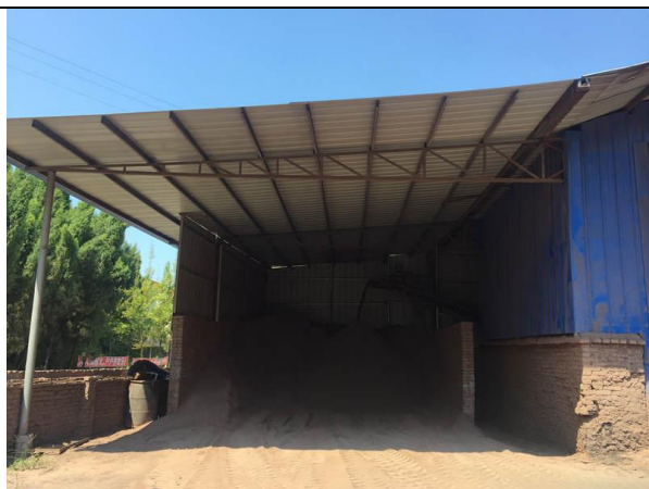
陈化库三面围挡+彩钢瓦顶棚
